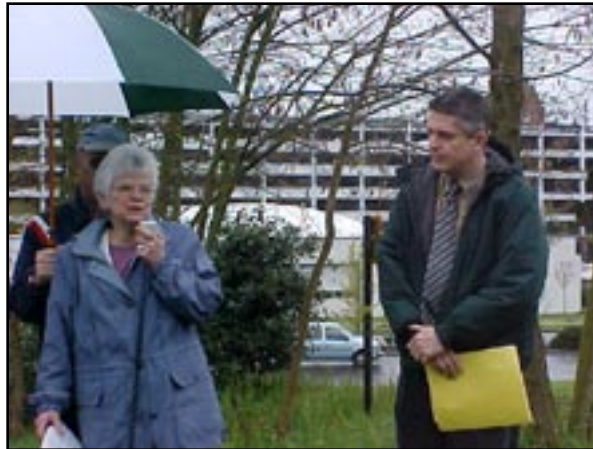
Sister Pat McMillan of the Catholic Community Services and President of Bremerton City Council, Daren Nygren, break ground on new shelter for homeless men.
